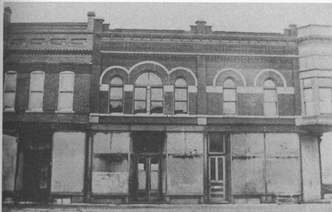
Note the architecture and the beautiful design of the building on the corner of Main and 4th Street.
